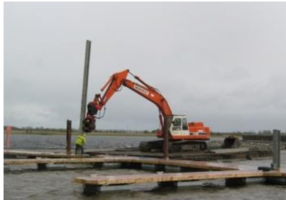
Figure 3-12: Pile Installation
