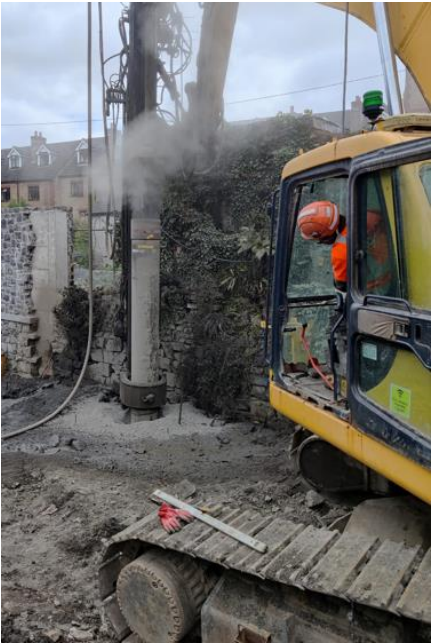
Figure 3-15: Core Drilling Attachment for round Jetty Piles
